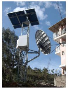
Figure 3: The La Encanada infocentre, Peru has solar panels to generate electricity and a satellite for connectivity. Photo: Practical Action / Jaime Soto.
